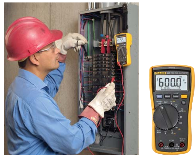
Figure 1-11 Testing for the presence of voltage.
