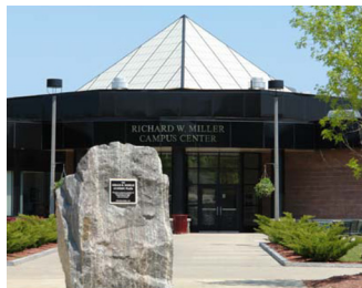
2002 Construction, Campus Center Addition
