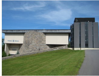
1960's and 70's Construction, Wicks Hall and Faculty Office Building
