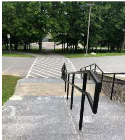
Figure 3.8: Stairs and Walkways Existing Payson Hall towards Rushton Hall
