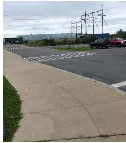
Figure 3.10: Roadway from Lot 4 to Athletic Center
