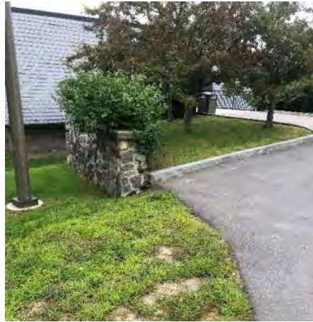
Figure 3.4: Retaining Walls and Landscaping at Chaney Diner Center
