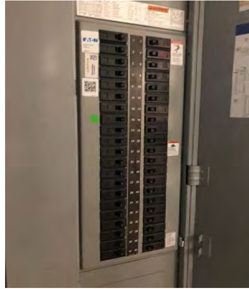
Figures 22: Upper Level Electrical Closet – Typical Branch Panelboards
