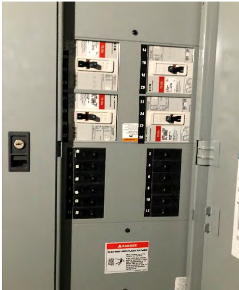
Figures 22: Upper Level Electrical Closet – Typical Branch Panelboards
