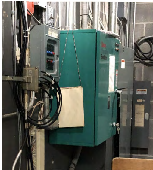
Figure 25: Transfer Switch
