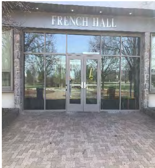
Figure 50: Upper Level Entrance
