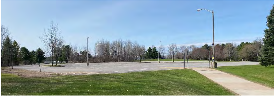
Parking Lot #7 – Proposed Ground Source Heat Exchanger Location
