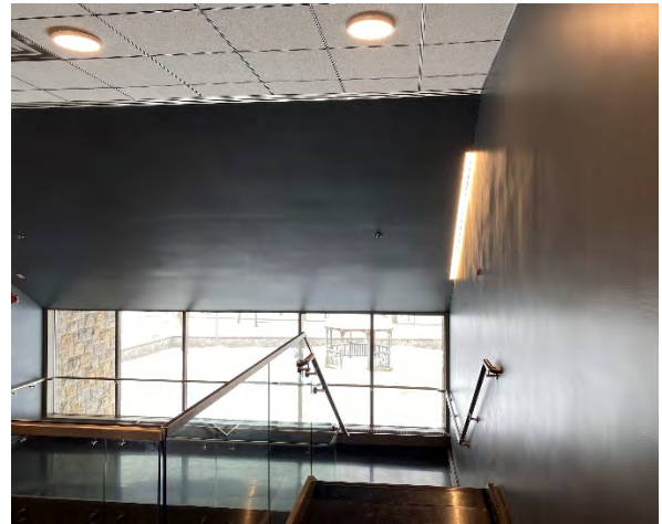
Figure 10: Upper Level Air Handler is Located above Communicating Stair
