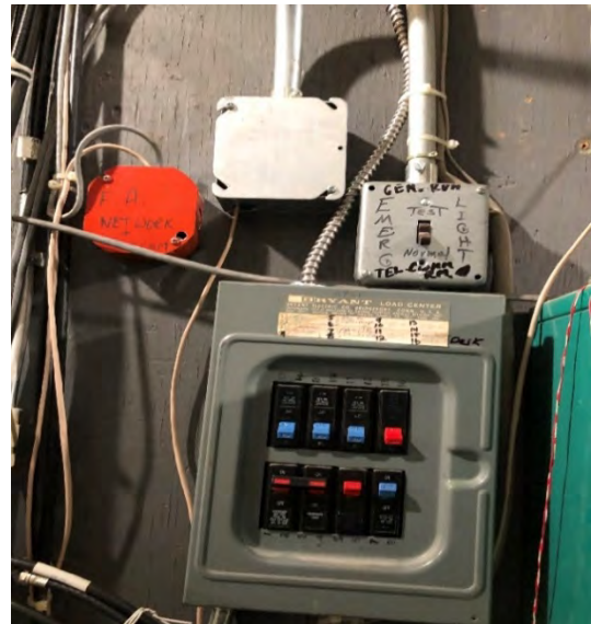
Figure 26: 8-Circuit Load Center
