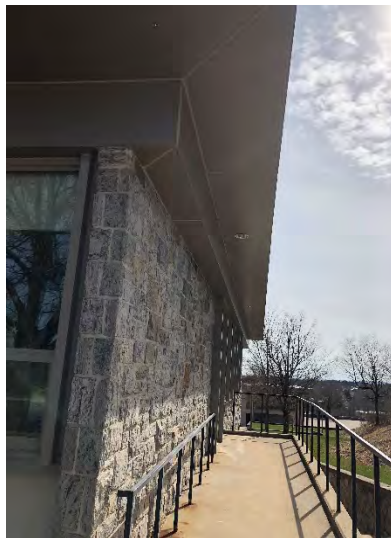
Figure 52: North Exterior Building Lighting
