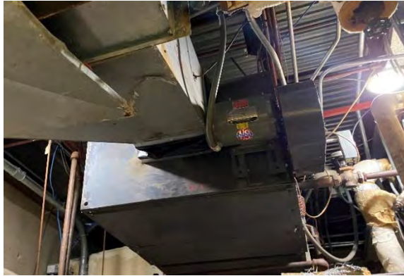
Figure 5: 1,560 CFM Lower Level Vent. Unit
