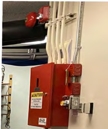
Figure 34: Clean Extinguishing Agent System
