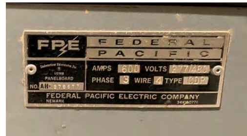
Figure 21: Panelboard Nameplate
