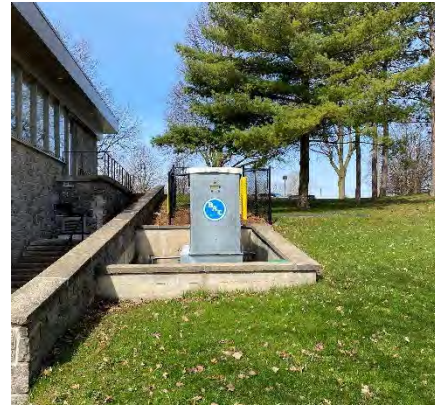
Figure 4: Cooling Tower adjacent to French Hall
