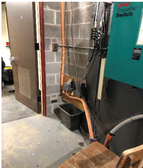
Figure 48: Utility Room Light Switch
