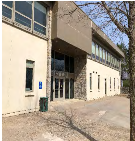
Figure 51: Lower Level Entrance
