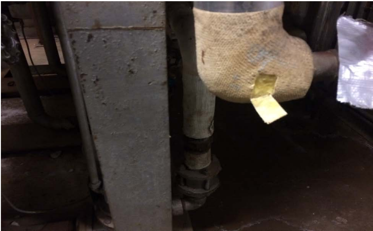
PHOTO #5 - Photograph of typical canvas wrapped elbows with fiberglass insulation in Mechanical Room of Wicks Hall. The canvas wrap was determined to be non-ACM.
