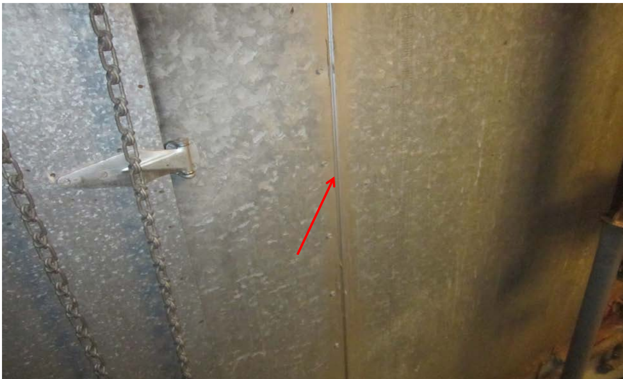
PHOTO #4- Photograph of asbestos-containing seam sealant on air handling unit in the Mechancial Room in MacArthur Hall.
