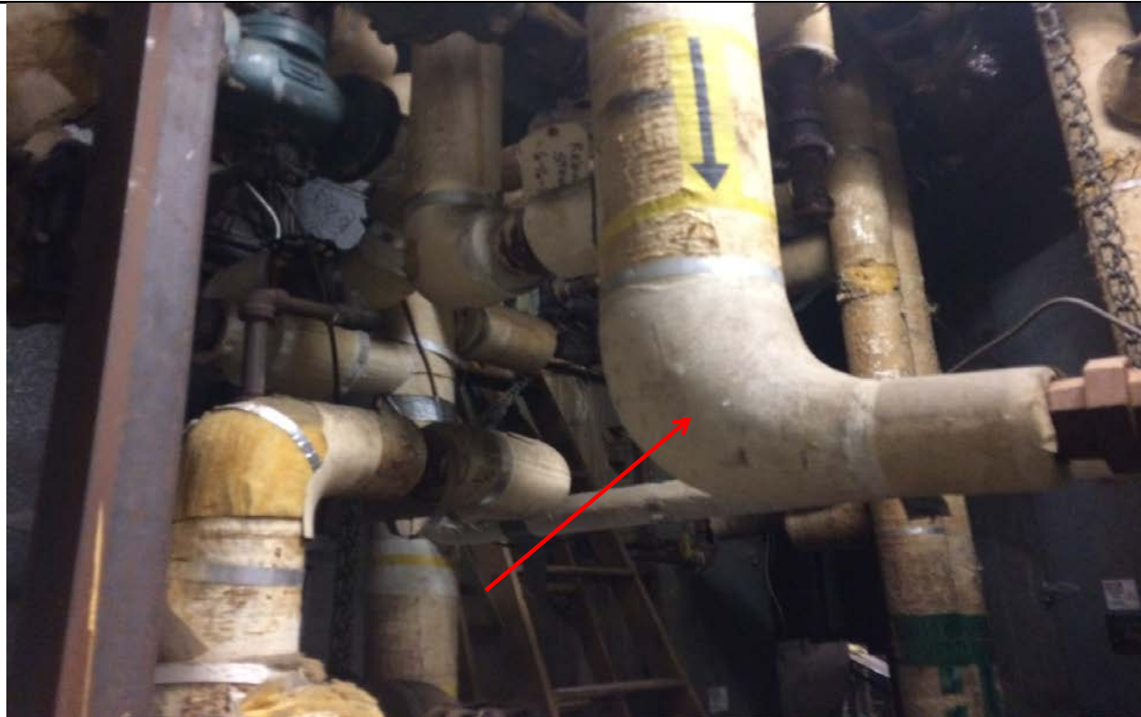
PHOTO #6 - Photograph of the a typical mudded joint fitting insulation in the Mechanical Room of Wicks Hall. The mudded fitting insulation was determined to be non-ACM.
