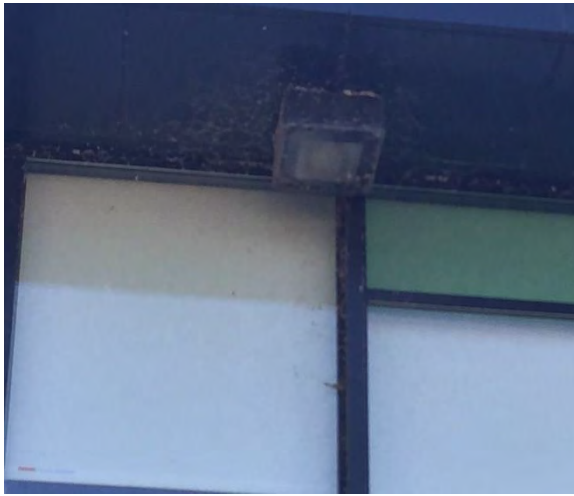
Figure 30: Wicks Building 2008 HID Luminaires Under West Roof Overhang
