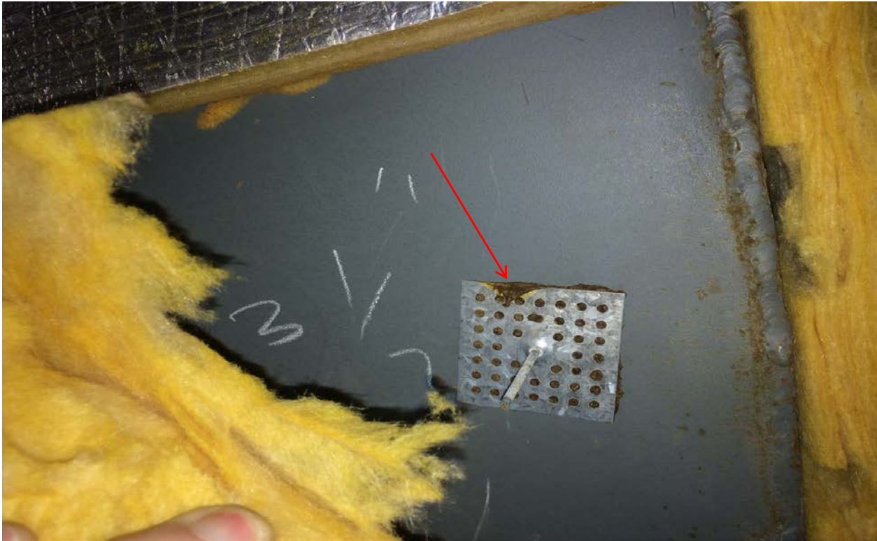
PHOTO #2- Photograph of asbestos-containing stick pin mastic on ductwork in the Mechanical Room of Wicks Hall.
