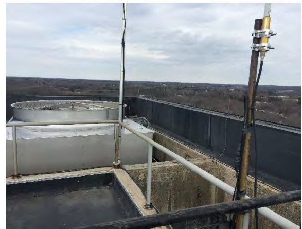
Figure 4: Cooling Tower on Roof of MacArthur Hall
