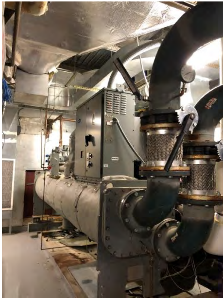
Figure 3: 325 Ton Water-Cooled Chiller in Penthouse
