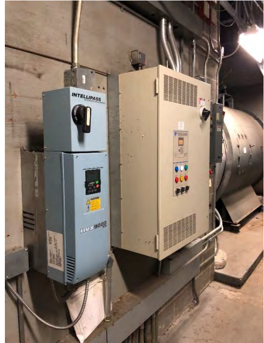
Figure 8: Speed drive for AC-2
