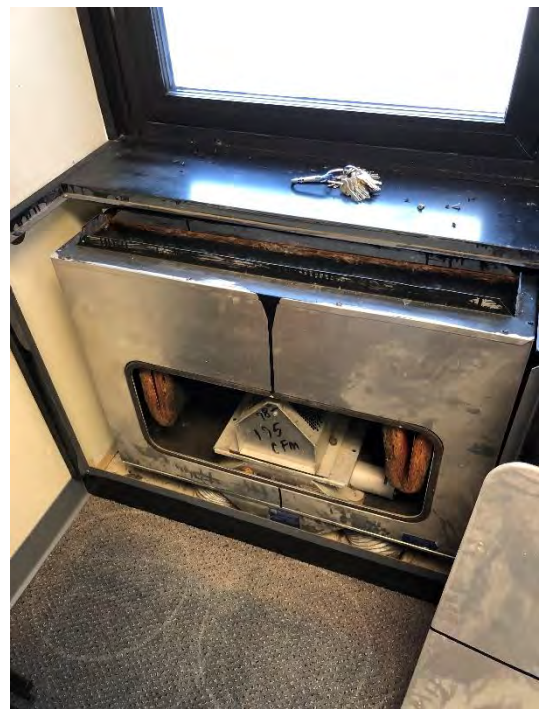
Figure 6: Existing dual duct box
