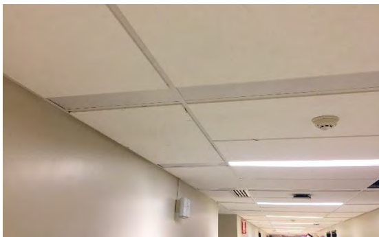
Figure 21: Wireless Access Point in Corridor
