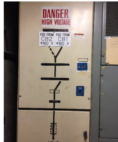
Figure 12: Service Entrance Transfer Switch
