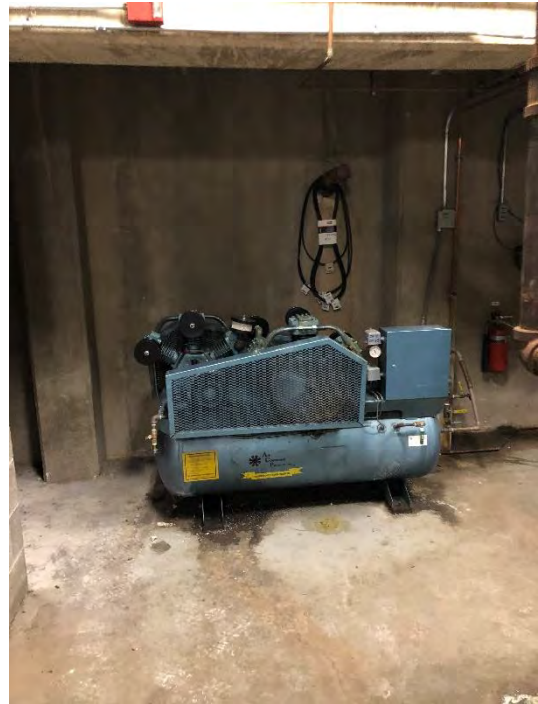
Figure 10: Control Air Compressor
