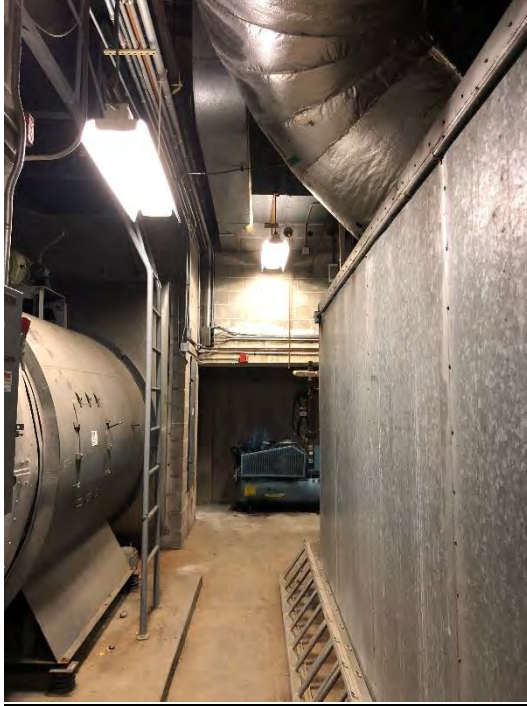
Figure 7: AC-2 with remote return fan
