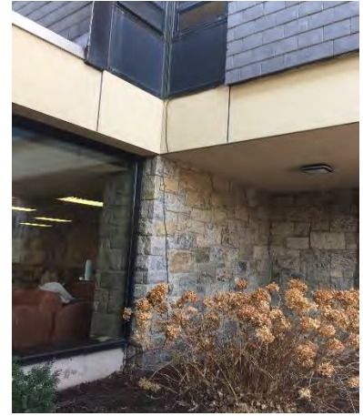
Figure 40: LPS Down Conductor
