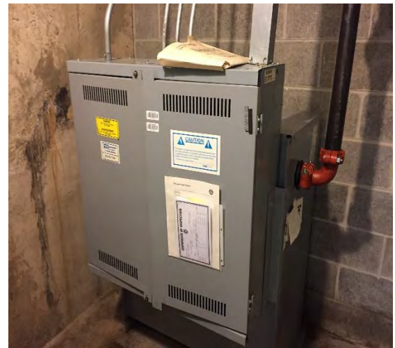
Figure 37: Wicks Elevator Machine Room
