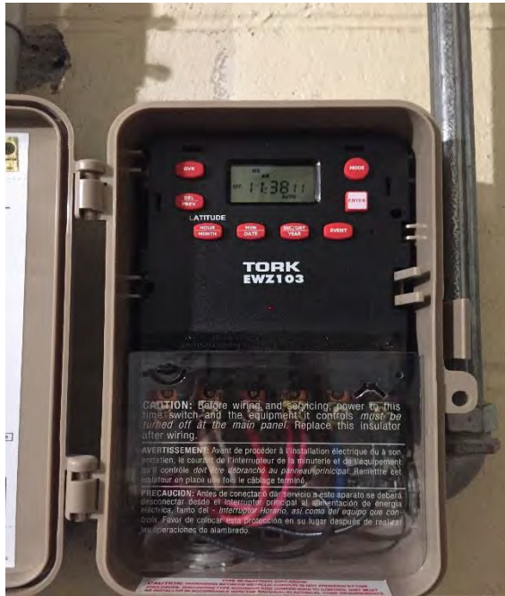
Figure 34: Exterior Lighting Time Clock
