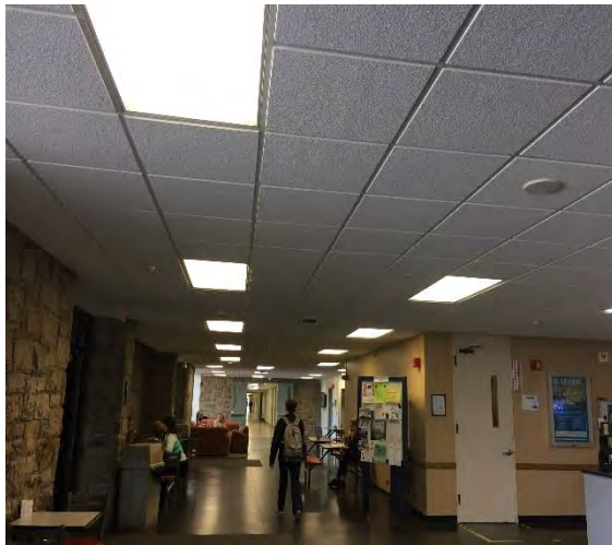
Figure 26: Lobby Fluorescent Troffer
