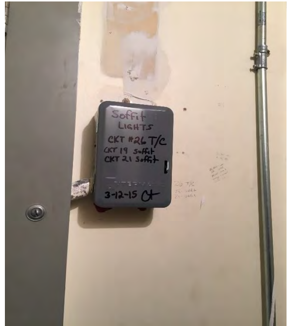
Figure 35: Exterior Lighting Time Clock
