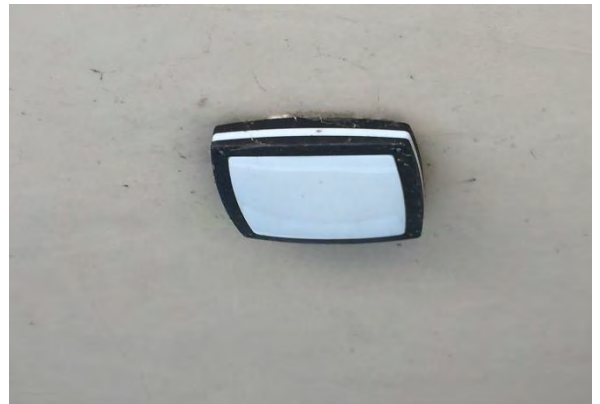
Figures 33: Side Entrance Canopy Luminaires Appear to be Replaced with LED Type
