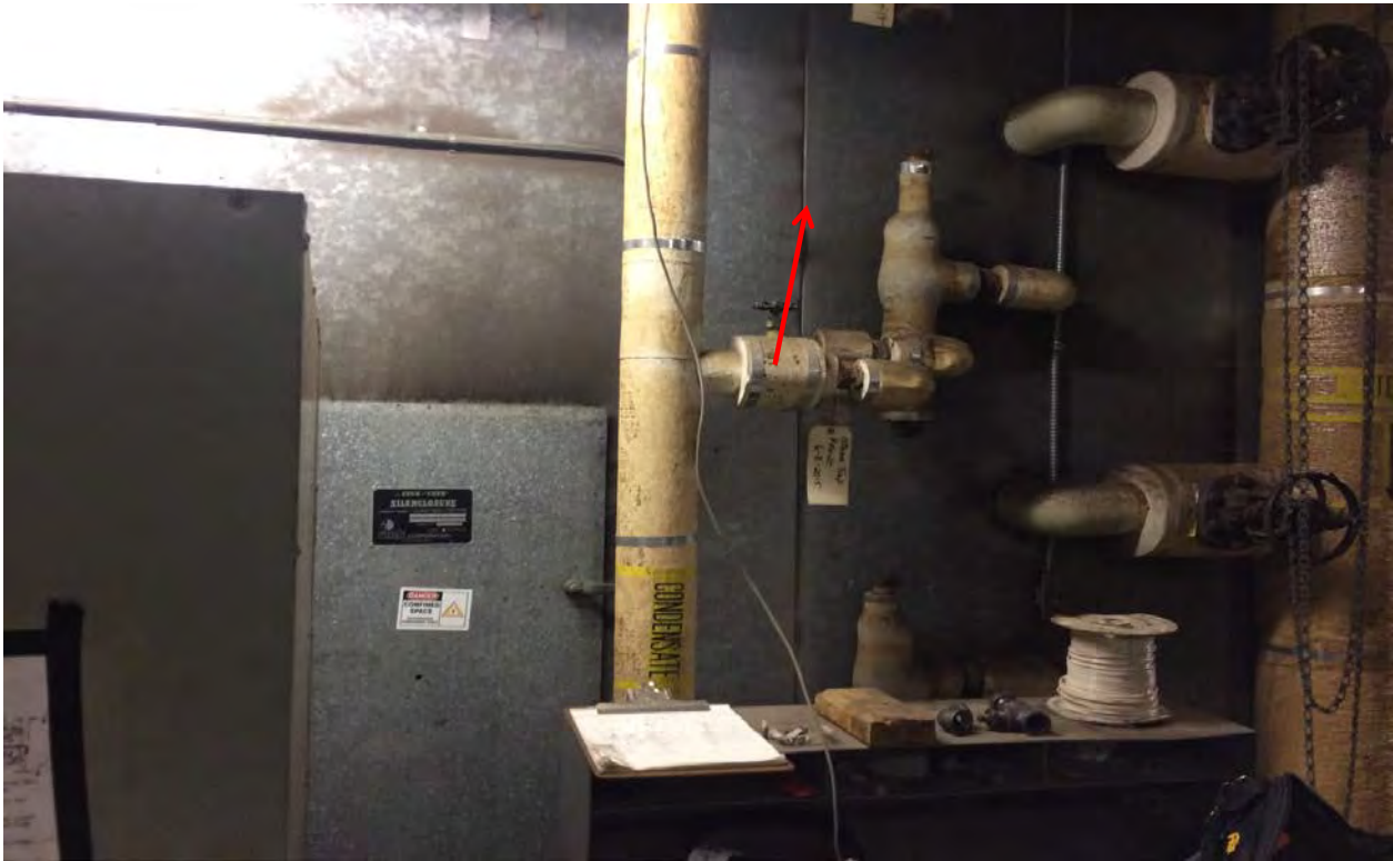
PHOTO #1- Photograph of asbestos-containing seam sealant on air handling unit in the Mechanical Room of Wicks Hall.
