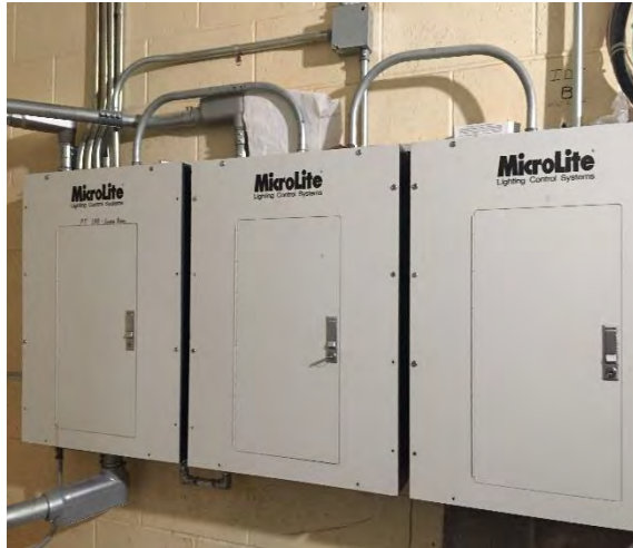
Figure 28: MicroLite Lighting Control System
