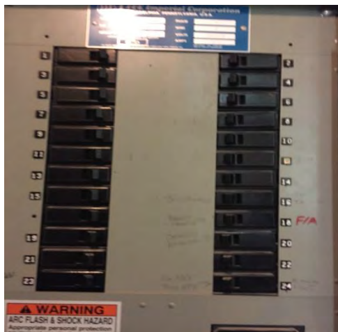
Figure 13: Typical Branch Circuit Panelboard
