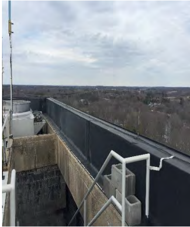
Figure 38: LPS Air Terminals
