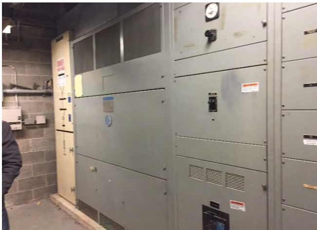
Figure 11: Electrical Service Entrance Switchgear
