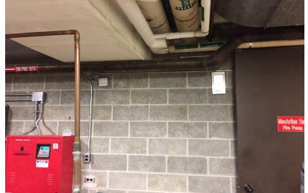
Figure 16: Water Line Over Inverters
