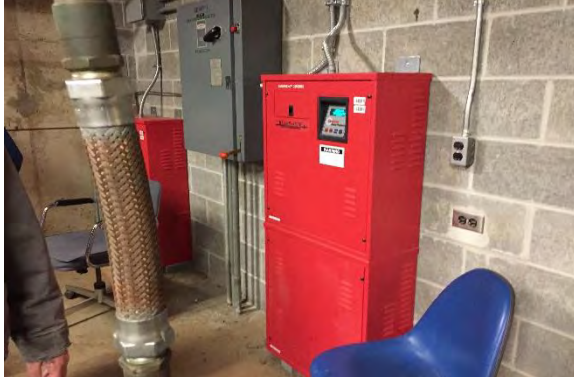
Figure 15: Emergency Lighting Inverters
