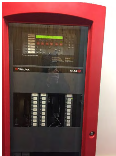
Figure 17: Fire Alarm Control Panel
