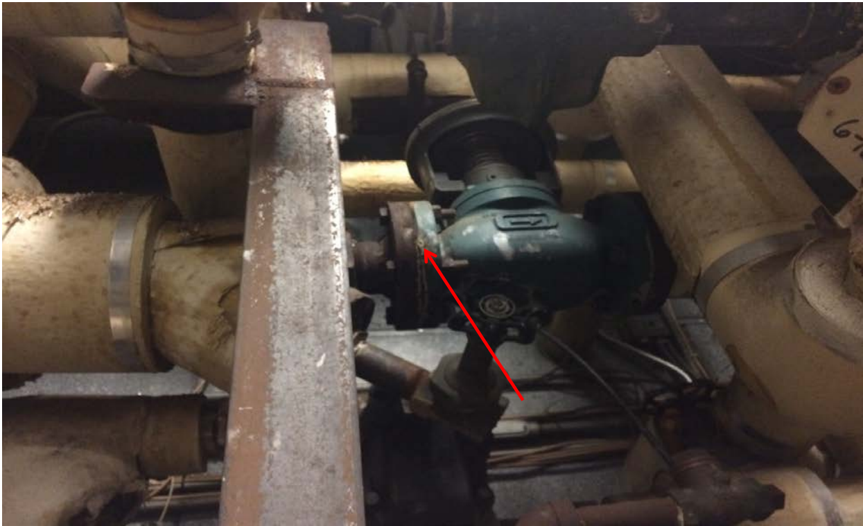
PHOTO #3 - Photograph of a typical flange, the gaskets associate with the flanges in Wicks Hall are asbestos-containing.
