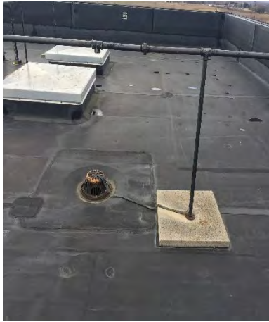
Figure 39: Metal Bonded to LPS
