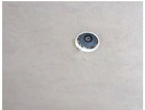
Figures 32: Original (Recessed Can Type) Canopy Luminaires at the Building Entrance
