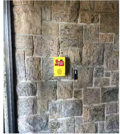
Figure 25: Card Reader & Emergency Station
