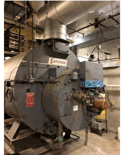
Figure 2: Existing Steam Boiler
