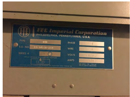
Figure 14: Panelboard Nameplate
