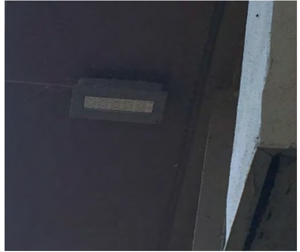
Figure 31: MacArthur Building LED Replacement Luminaires Under Front Roof Overhang
