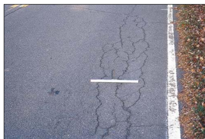
Figure 3: Fatigue (bottom-up) Cracking
