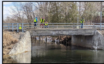
Figure 4: Fish Creek Bridge
