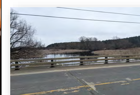
Figure 7 Black Creek Down Stream
