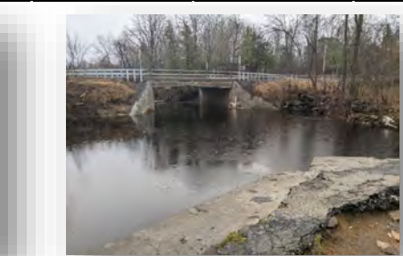
Figure 10 Upstream towards bridge
