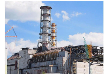
Above Right – Figure 9: The famous sarcophagus constructed over reactor unit 4 to help contain the spread of radioactive material
