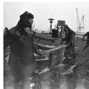
Above Right – Figure 7: Chernobyl Liquidators removing contaminated debris from the roof of the reactor unit building
