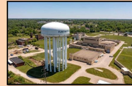
Figure 3 – Flint, MI's water treatment plant
