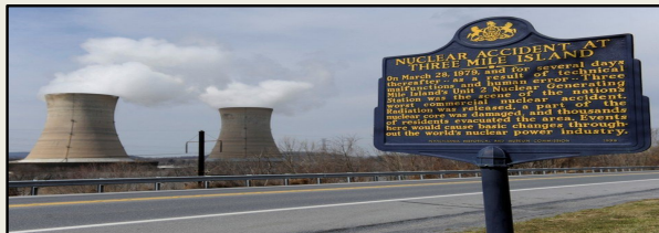
Figure 4: Cooling Towers Now
