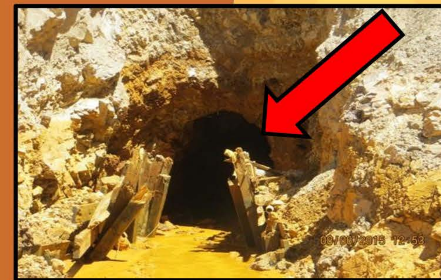
Figure 5. Plug entrance of the Gold King Mine Spill (flickr, 2015)
